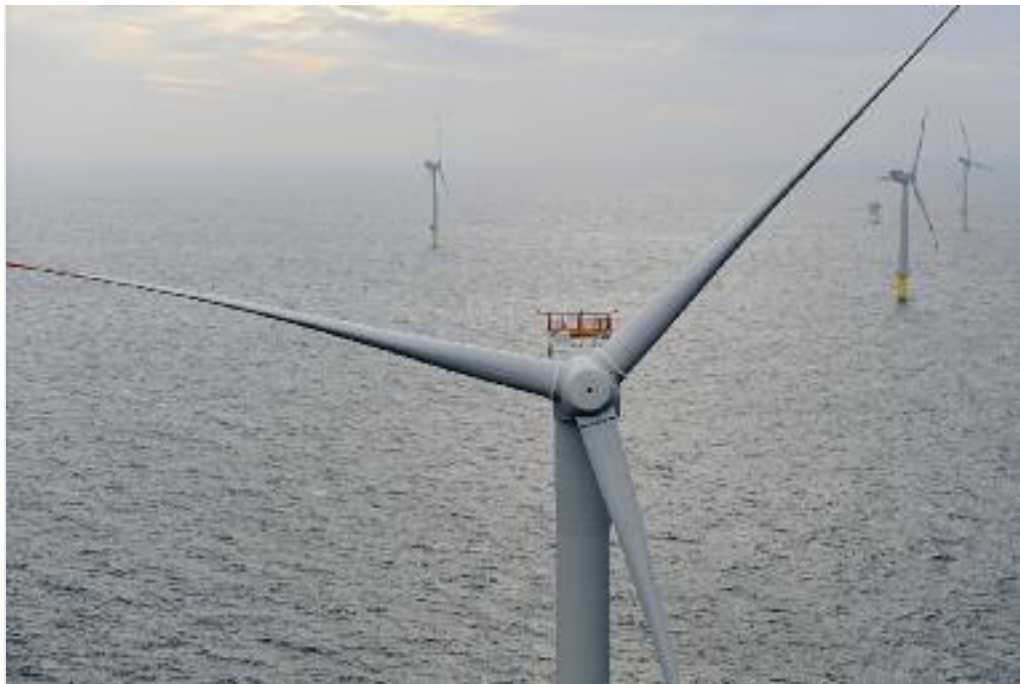
Offshore-Windpark in der Nordsee An offshore wind farm in the North Sea
