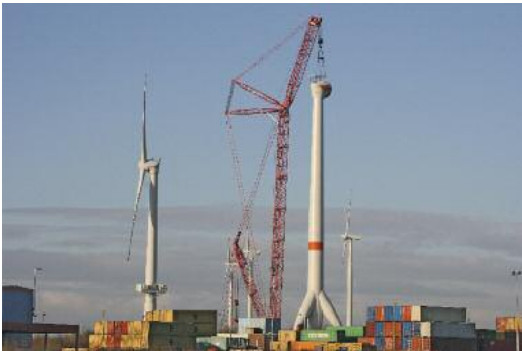
Montage von Tripod-Windkraftanlagen Installing wind turbines on tripod foundations
